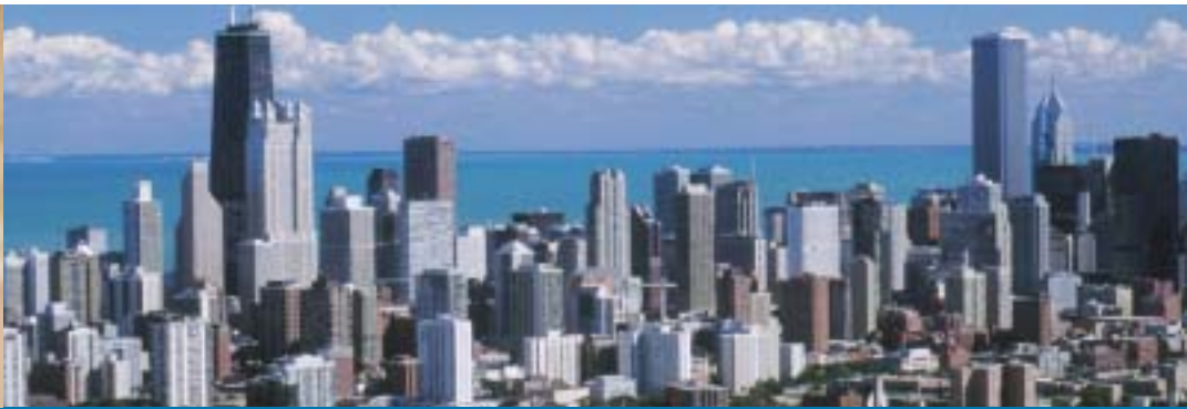
Aerial view looking East – City of Chicago/Peter J. Schulz
